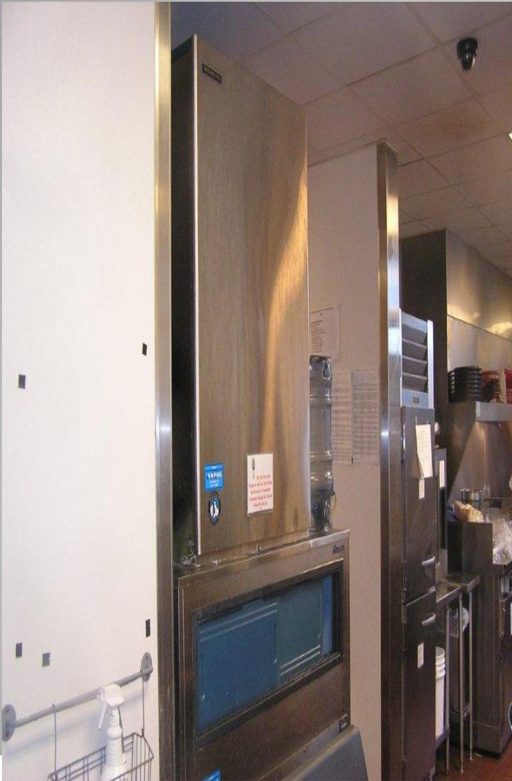
**Ice machine gets ice from the bottom making sure that the ice in the bin is always fresh. We have the compressor on the roof to keep the heat out of the kitchen and it is highly energy efficient**
