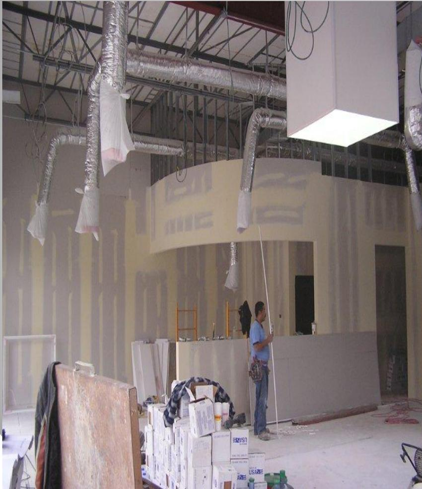
**The Skylights under Construction. Each skylight is 4X4x9 & has 4 mirrors that are 9 feet by 4 feet wide.**
