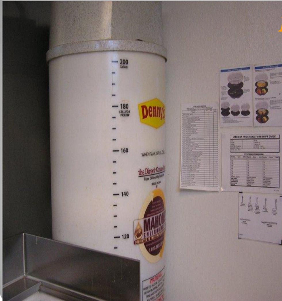
**The recycling vendor comes on a weekly basis and removes the oil through the wall with a vacuum hose hookup at 3AM not disturbing our business.**
