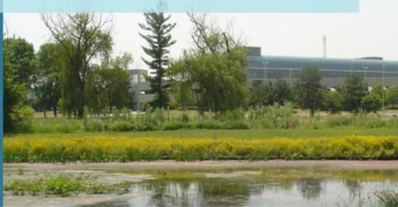
A native buffer is a strip of native vegetation around a stormwater detention pond. Adding a native buffer can enhance the function and appearance of a detention basin.
